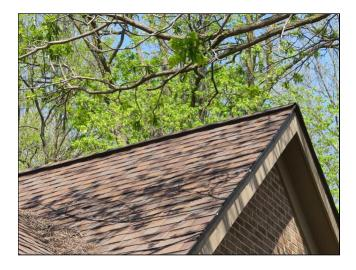
◆ Areas where the roof slopes towards the structure are prone to water intrusion and ice damming and should be monitored closely for leaks and maintenance as needed. Leaks might not be apparent except when actually occurring. Because of the nature of construction, important portions of the flashing are concealed from view
