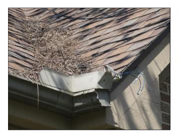
◆ The valley shingles were not all trimmed according to roofing specifications. The upper corner of each end shingle should be trimmed on a 45 degree angle to direct water into the valley and discourage water flow under the shingle surface. In many cases, no leaks occur, but as a precaution, we advise having corrected to help shed water.
